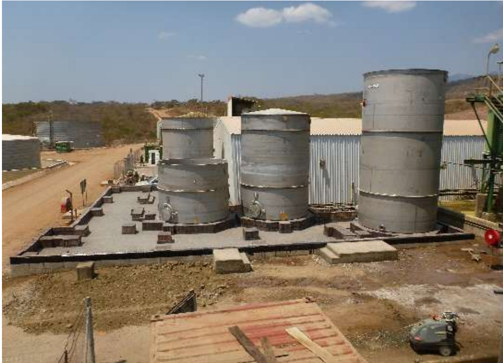
Pad installed while Skids being fabricated
