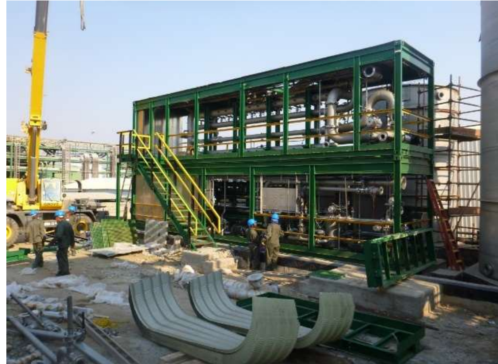
Skid installation completed within weeks
